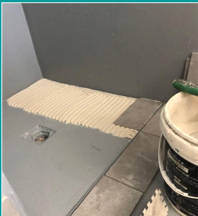
Figure 8: Shower recess tiles being laid on the sand-cement bed
